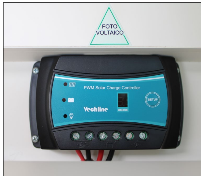
Solar charging controller for the optional solar power system (sample illustration)
