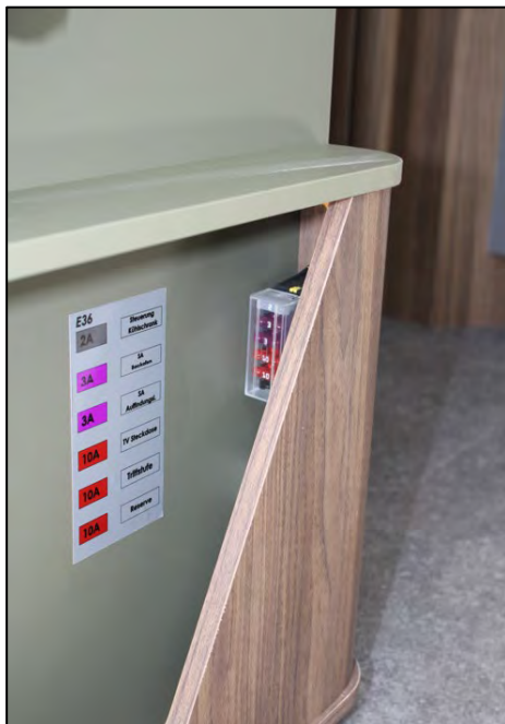
Additional fuse holders in the entrance area (sample illustration)
