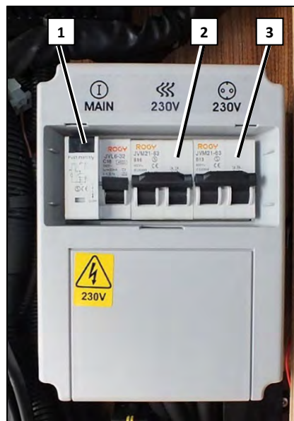
230-V protection with RCD (sample illustration)
