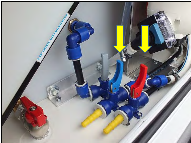
Drain valves for cold and hot water (sample illustration)
