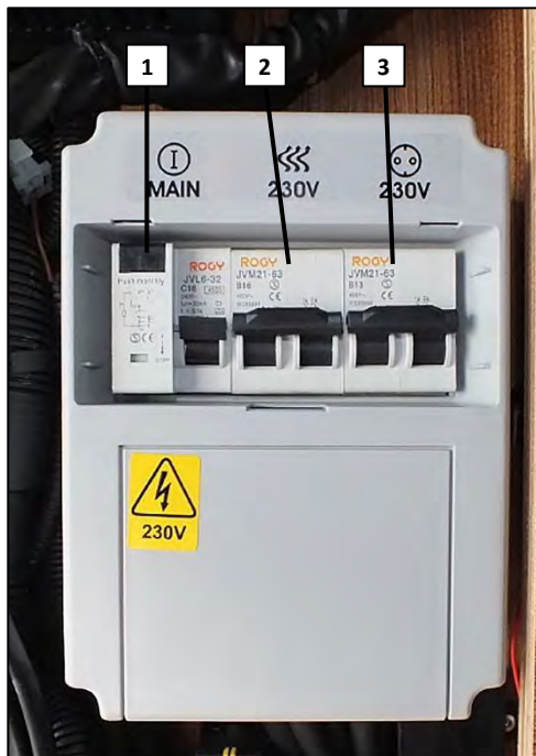
230 - fuse with RCD (sample illustration)
