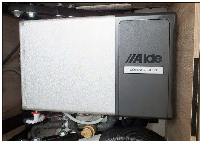
Gas powered ALDE Compact heating system (sample illustration)
