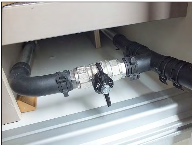
Valve for activating the waste water tank heating (sample illustration)
