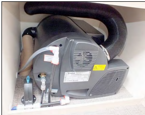
Gas powered TRUMA Combi heating system (sample illustration)
