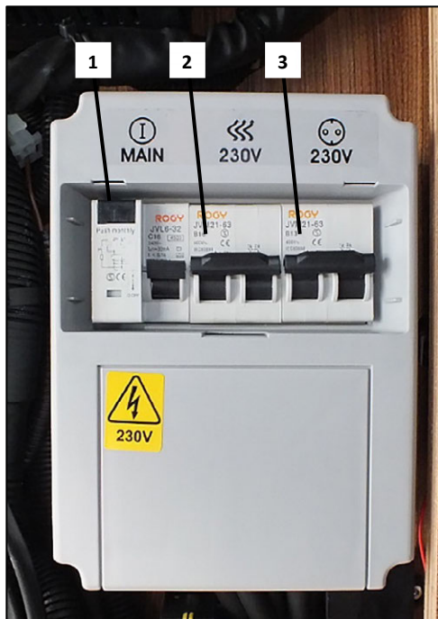
230 V fuse with RCD (sample illustration)
