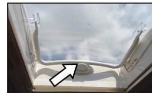
Closing the miniature opening skylight
