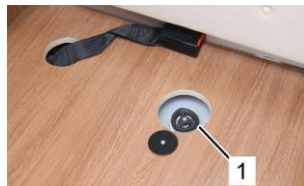
Drain cock fresh water tank
