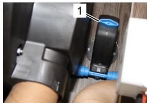
Safety/drain valve: FrostControl
