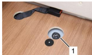
Drain cock fresh water tank
