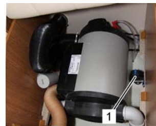
Safety/drain valve: FrostControl
