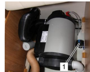
Safety/drain valve: FrostControl
