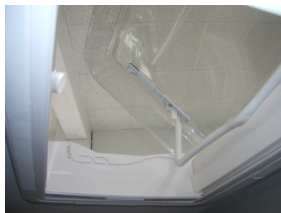
Roof hatch open
