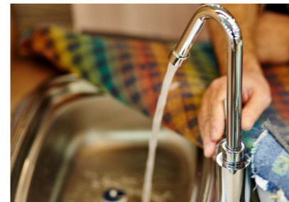
Correct installation of the hydraulic systems.
