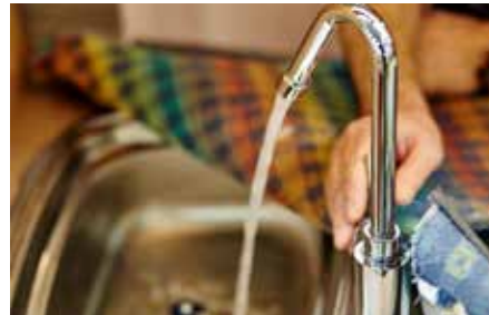
Correct installation of the hydraulic systems.
